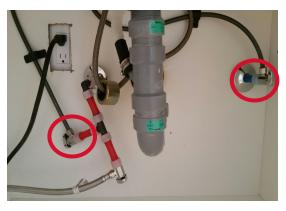
Hot and cold water shut-off for the kitchen sink
