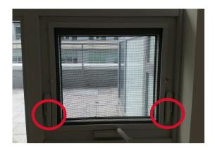
Please make sure both window latches are completely in the upright position before you use the handle to open the window.
