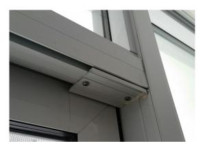
Take care not to pull Balcony Slider Doors to hard so as to hit the stop and dent the door.
