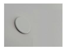
You will find fire sprinklers located throughout your suite as part of the Fire Code. Do not tamper, remove or paint these covers as it may set off the sprinkler system.
