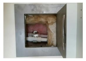
Main water shut-off in Main Bathroom
